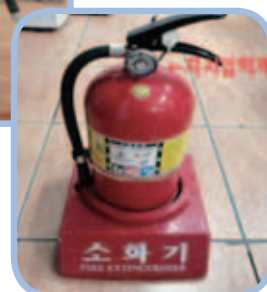
Stored-pressure type (having a pressure gauge)
